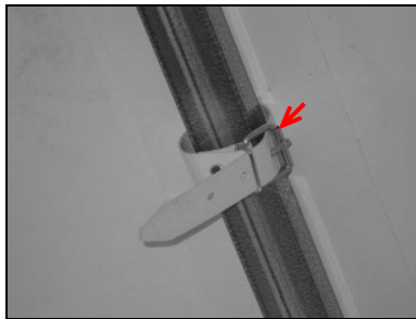
Tensioning belt on traverse roof beam
