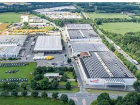
Production facility Herzlake (Germany)
