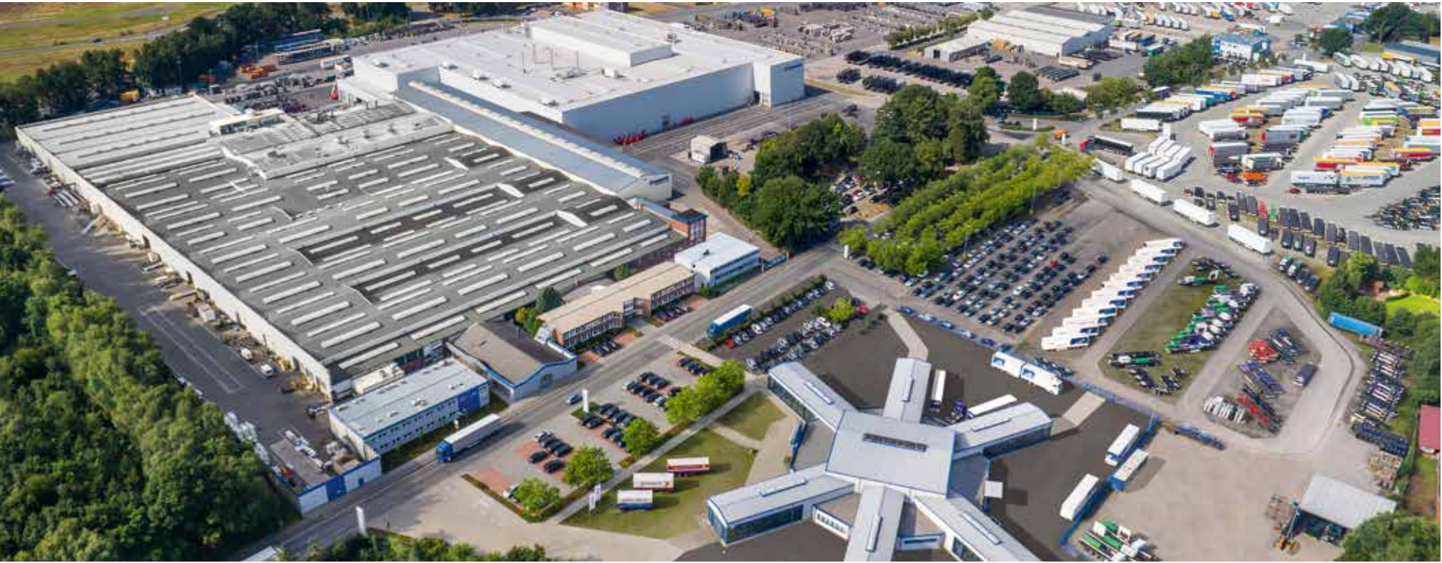
Production facility Wertle (Germany)
